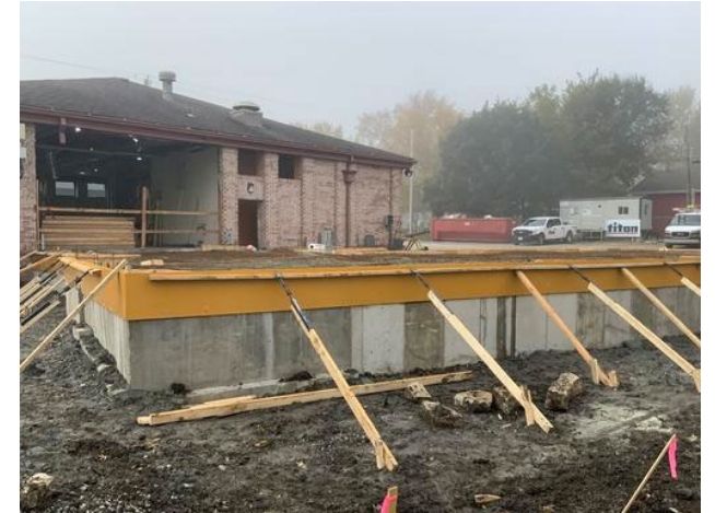
View of new addition foundation from south and west, prior to slab concrete pouring
