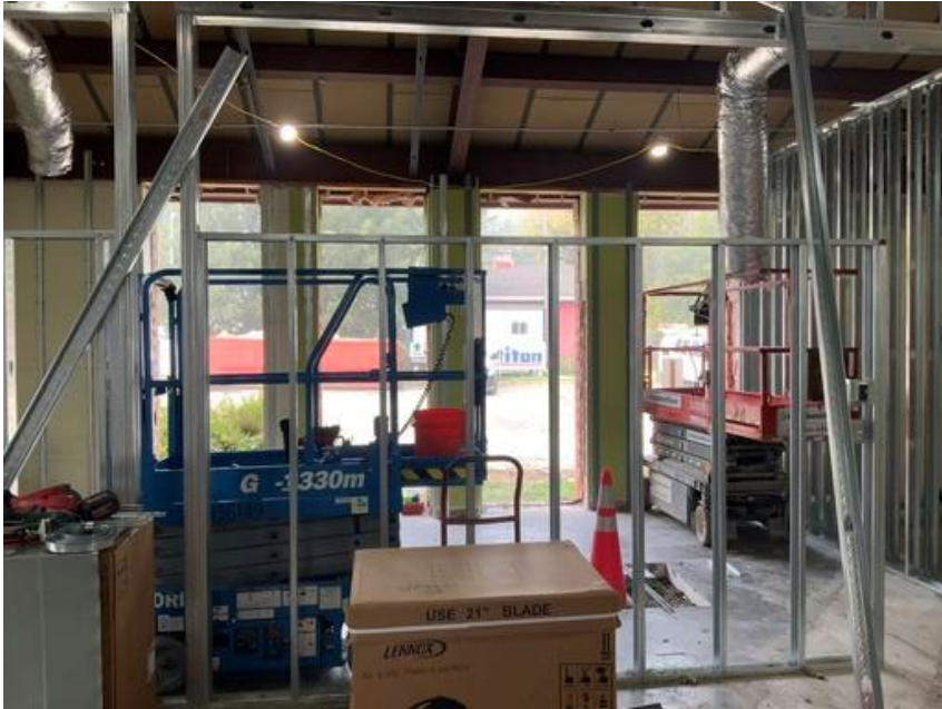
View of new window openings in future conference and study room; walls framed and HVAC ductwork hung
