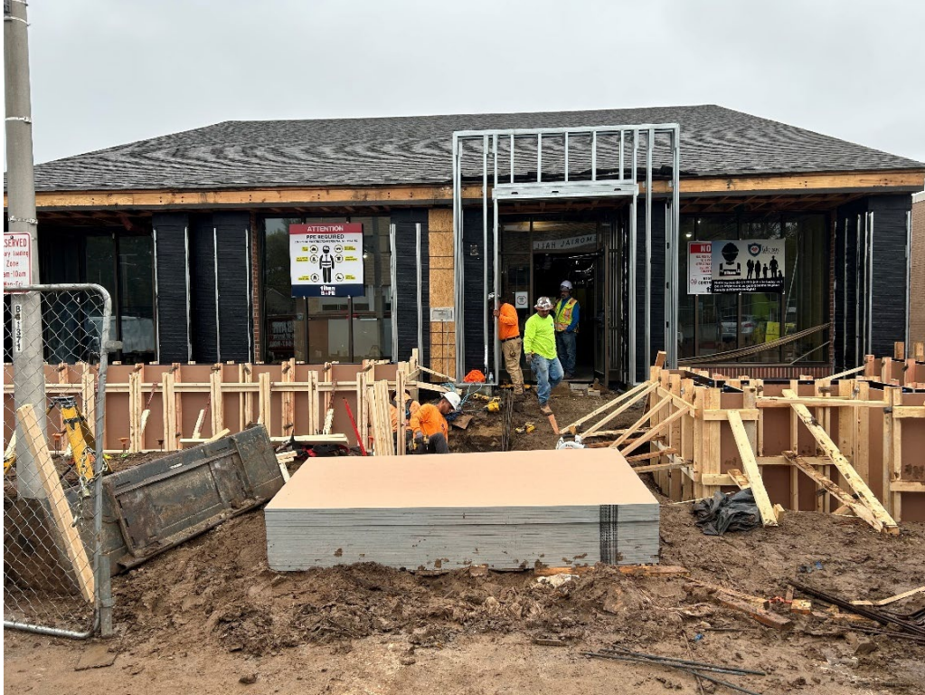
View of front of building. Demolition of fascia and soffits, new façade framing started, and entryway footings poured.
