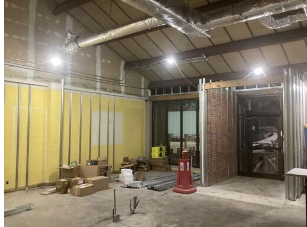
View of northwest, looking towards kids area. Interior wall framing begun, HVAC run overhead, concrete poured over new electrical.
