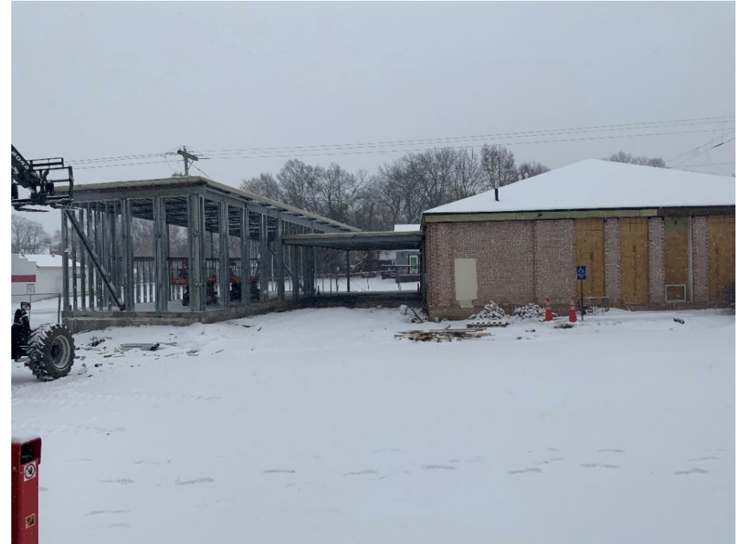
Exterior view of the west side, showing the new addition steel structure framework connected to the existing brick building.
