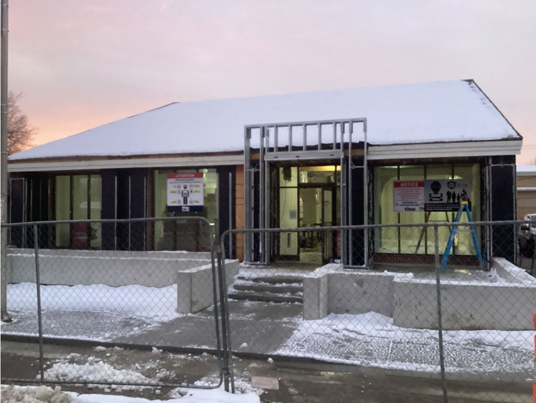
View of the front. Concrete poured: ADA ramp, stairs, seating area pad, and new sidewalk.
